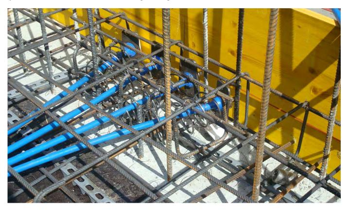
20.1 - Application of unbonded anchorages
