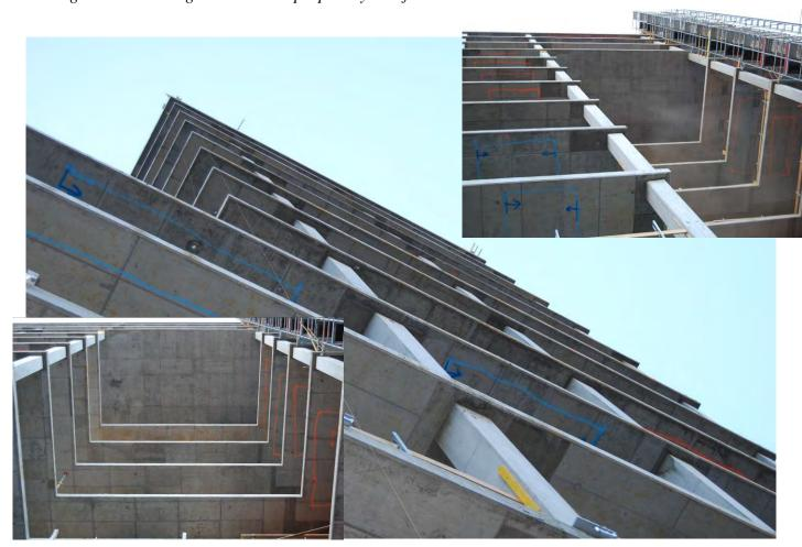
Post-tensioning is very favourable in the construction of rectangular slabs with 8-12 m long sides. The design of these slabs requires the use of mesh of single strand cables from unitary strands, having steel reinforcement sections of: 139 mm<sup>2</sup>, 150 mm<sup>2</sup> and 165 mm<sup>2</sup>.
