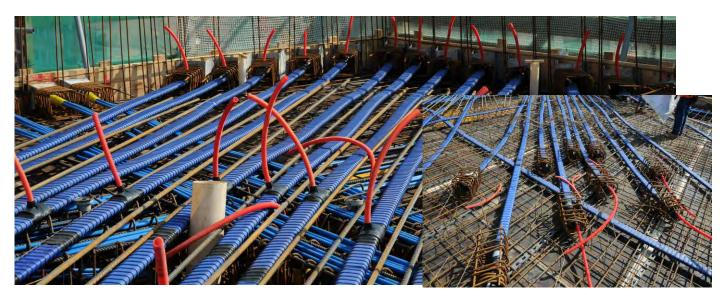
The bonded application is surely the easiest one, since it is protected against corrosion by the cement grouting that is a barrier against the strand oxidation by guaranteeing the discharge of air. The quality of grouting is the best warranty to the system durability, therefore the sealing completes the protection of the anchorage over time and its importance increases together with the anchorage exposure to corrosion.
