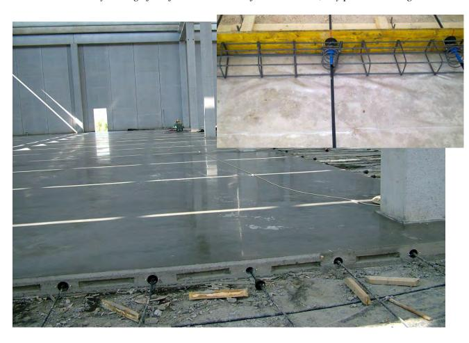
This application is used when following modifications shall be needed by cutting the plate on the posttensioned structured.
