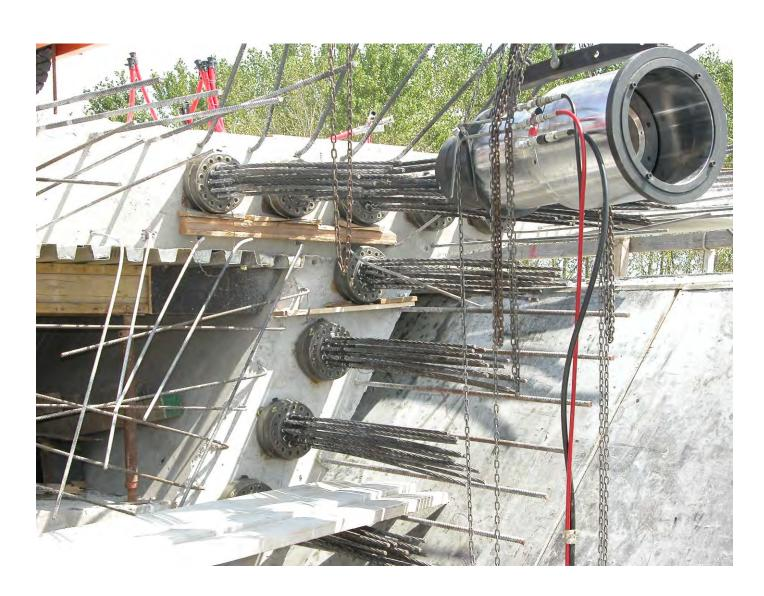
The "DD" series of jacks is available in four models which differ according to use characteristics. They are equipped with 10 m long flexible tubes and spanners of different sizes for all the types of bars from 26.5mm to 50mm. They are set up for automatic tightening. When the special spanner is inserted in the jack, the nut can be tightened keeping the bar under tension. This avoids the use of seatings and manual tightening operations.
