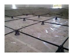
The post-tensioned system that is usually used for slabs can also be applied to carry out industrial floors, thus allowing the floor industry to also take advantage of this technology.
