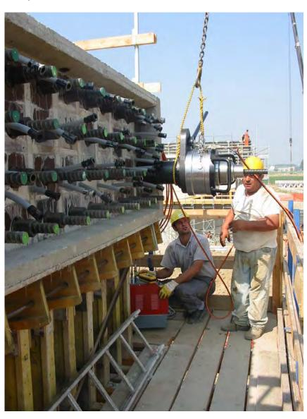
Bar tensioning of diam. 40 mm with DD2000KN jack and TTM250-A pump Page 159
