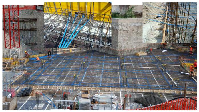
The unbonded application is surely the most performing one, since it is protected against corrosion by both a grease and a polyethylene barrier. It requires no grouting after tensioning but a very accurate infilling (sealing) of the heads. In this application the load will always remain totally concentrated on the anchorage, therefore the sealing completes the protection of the anchorage over time and its importance increases together with the anchorage exposure to corrosion.
