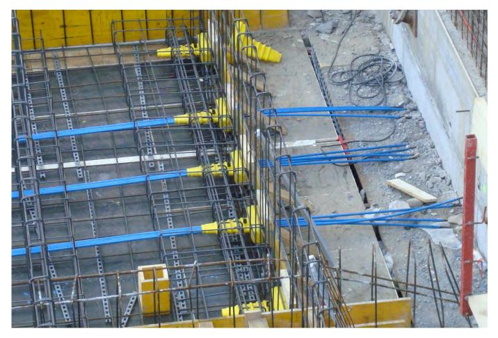
3.2 - "L" series bonded anchorages (Bonded post-tensioning)
