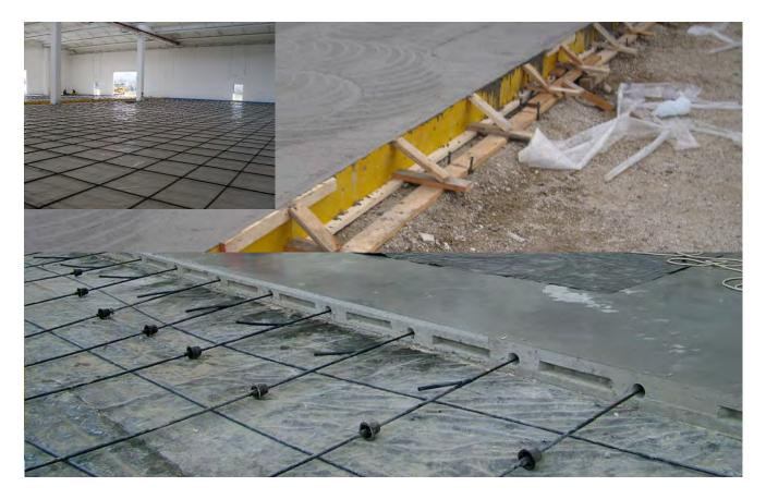
**1.6.2** Positioning of wire strands Wire strands are positioned in the middle of the plate thickness by means of spacers in order to make the applied stress more compact and even.
