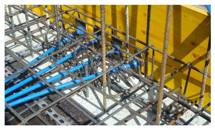
2.1 - Application of unbonded anchorages
