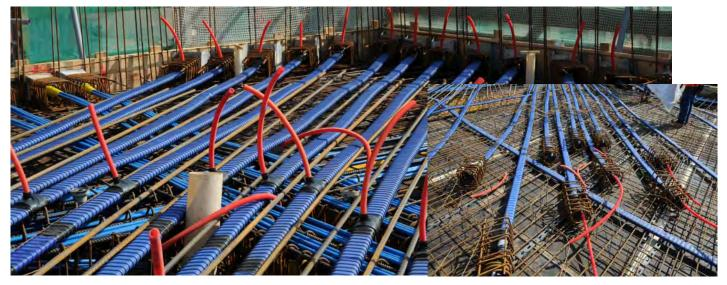
The bonded application is surely the easiest one, since it is protected against corrosion by the cement grouting that is a barrier against the strand oxidation by guaranteeing the discharge of air. The quality of grouting is the best warranty to the system durability, therefore the sealing completes the protection of the anchorage over time and its importance increases together with the anchorage exposure to corrosion.
