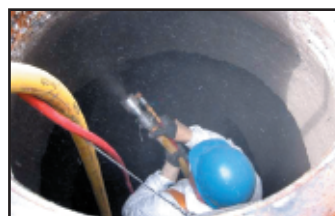
Manhole Sealing
